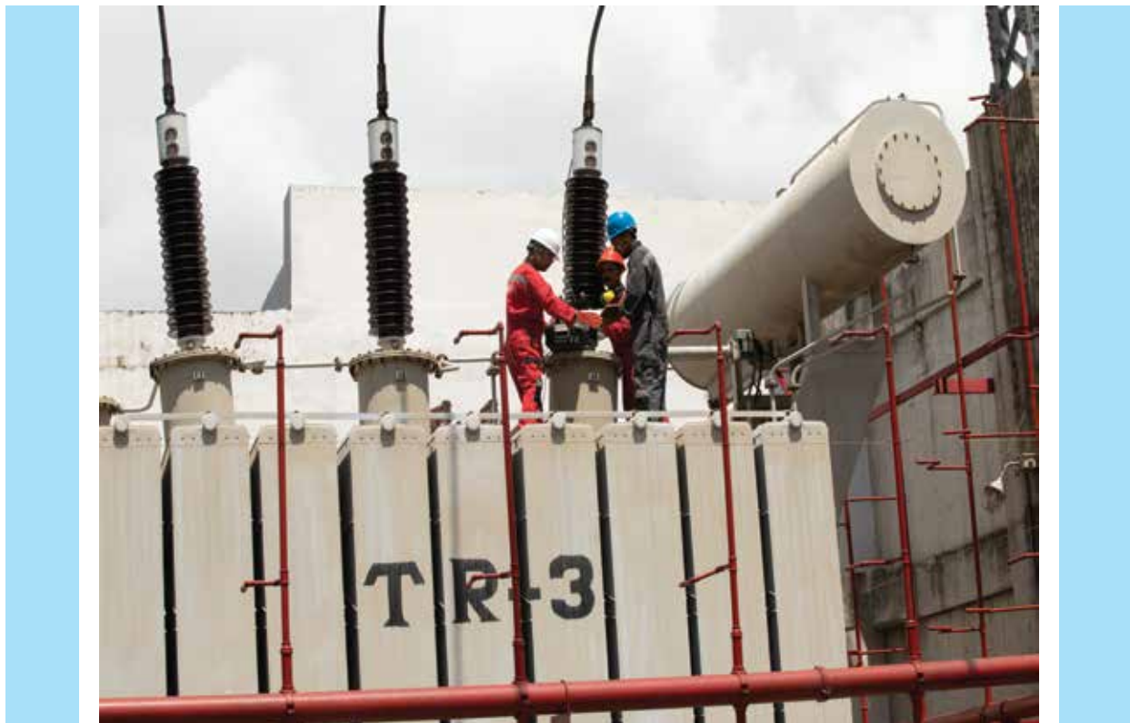
Kodda 150 MW Dual Fuel Power Plant, Gazipur.
