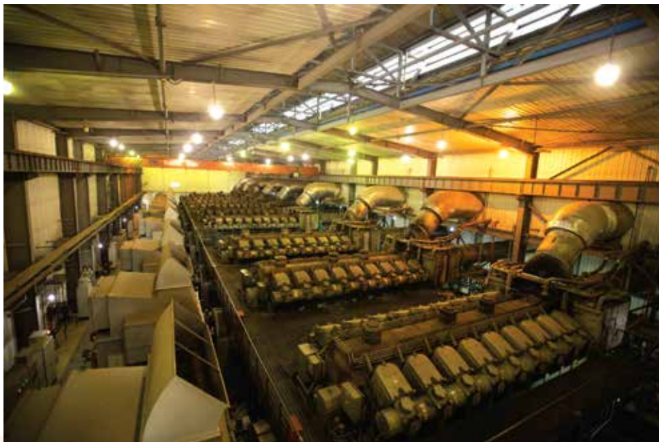
Engine Hall of Kodda 150 MW Power Plant at Kodda, Gazipur.
