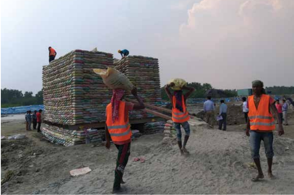
Pile Test work Mirsarai 150 ( \pm 10\% ) MW Dual Fuel Power Plant Project
