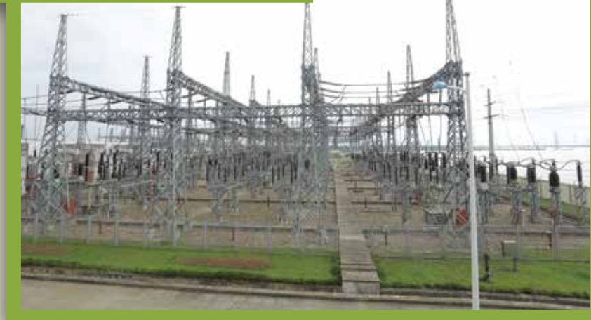
Koda 150 MW Dual Fuel Power Plant, Gazipur.
